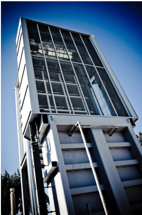
A GT power plant using carbon negative technology.
